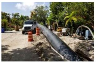
Construction of a new 7.5-mile redundant forced main sewer required two contractors using horizontal directional drilling (HDD) to install the 54-inch diameter HDPE pipe. Murphy Pipeline Contractors, Inc. (Jacksonville, FL) ran from the north while David Mancini and Sons (Pompano Beach, FL) came from the south. Both companies are contractor members of the Municipal Advisory Board, an independent, non-commercial adviser to the Municipal & Industrial Division of the PPI.
