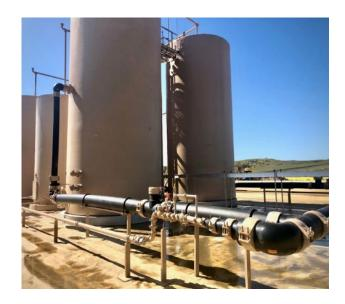
Permitted to accept up to 50,000 barrels per day (b/d) of produced water, the Crestwood Gondor Saltwater Disposal facility features two wells, two separators, two oil storage tanks, and 10 produced water storage tanks across nearly three acres. The project, which was constructed using both onsite installation and in shop fabrication, consisted of 12 inch and smaller HDPE pipe.
